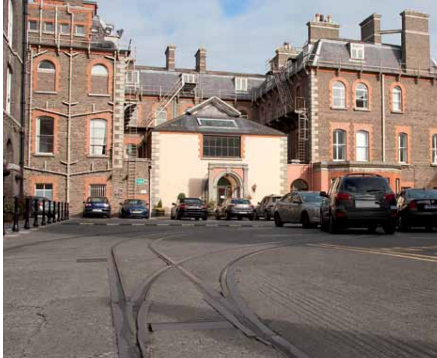
Tracks still lying in the roadways are a relic of the narrow-gauge goods railway which once served the 63-acre site. A tunnel, still in use, led them under the street outside
