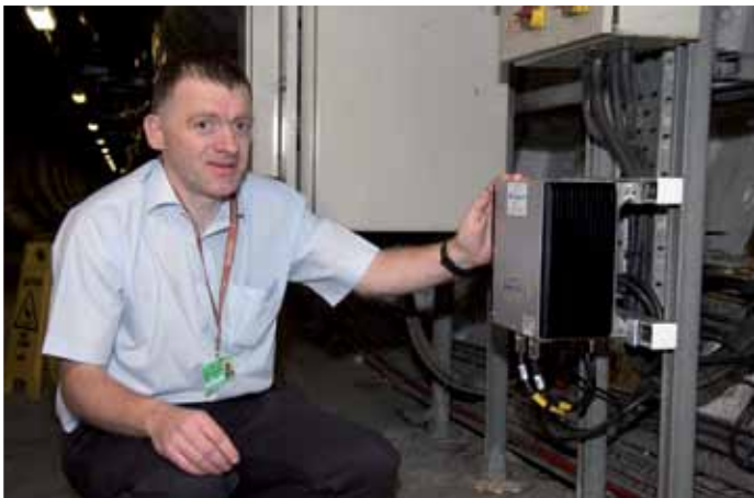
Clockwise from top left: the 'hot tunnel', built to carry steam-pipes beneath a main road which bisects the brewery site, which was one of the few areas not reached by the UHF Nexedge signal; an antenna installed within the tunnel as part of a coverage reinforcement system provided by PMR supplier BP Multipage; Dave Gerachty, service manager for BP Multipage, with the tunnel booster he installed, a bidirectional amplifier by the French manufacturer ETSA; and, on a wall outside, the pickup antenna which feeds the tunnel amplifier
